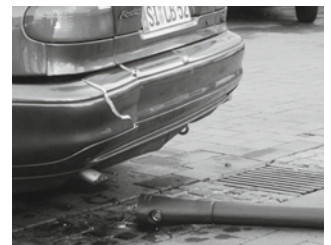
2 | Damaged bollard
