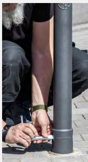
Bollards with junction pieces (3p-Technology) fit in the same ground shell.
