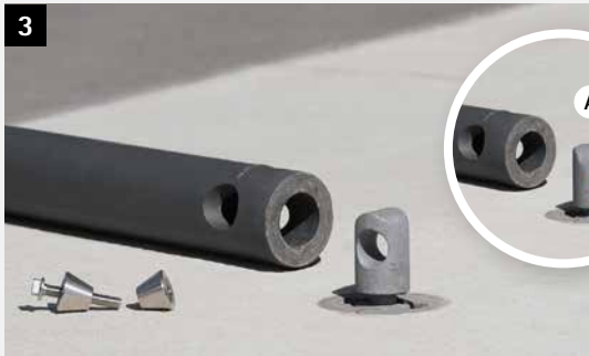
A) Insert a new junction piece in the ground shell and turn it by 90°
