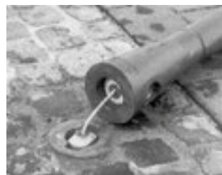
3 | Bollard system after damage
