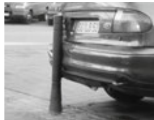
1 | Bollard before damage
