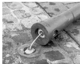
3 | Bollard system after damage
